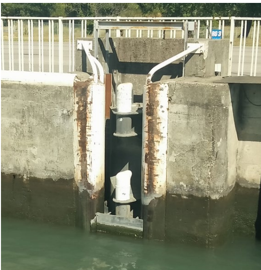
The double floating bollards in the large locks on the Rhone. When we learn that we can pass a rope to one single bollard at midship, everything becomes much easier.
